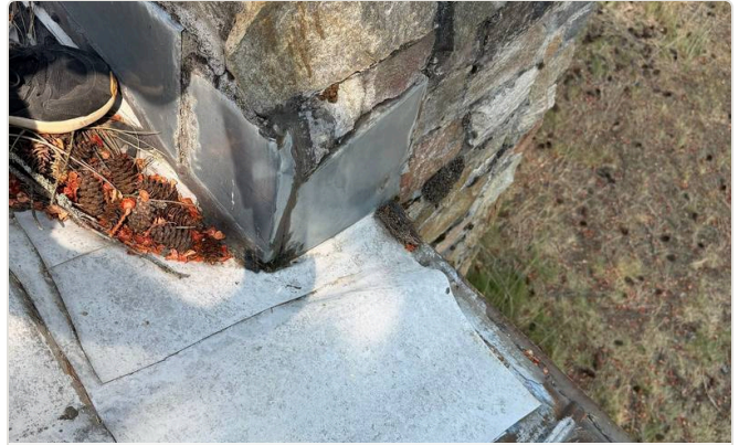
STONE CHIMNEY AND EXISTING COUNTERFLASHING (ALTERNATE B)
